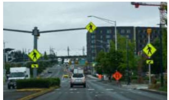
Figure 19. Crosswalk and RRFBs along Tukwila International Boulevard
