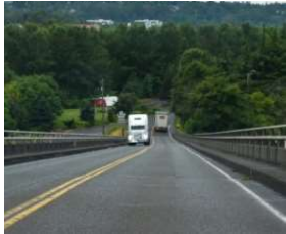
Figure 32. T-3 Corridor – S 129 th Street Bridge
