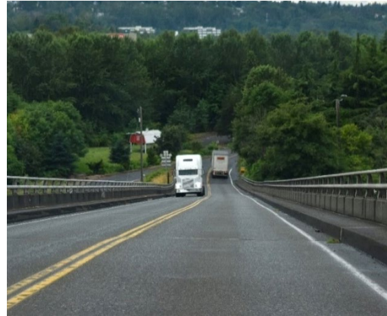
Figure 32. T-3 Corridor – S 129 th Street Bridge
