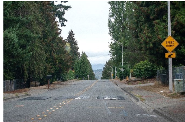
Figure 34. Speed Cushions in Tukwila
