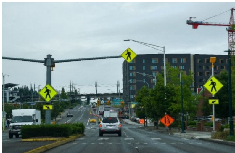
Figure 19. Crosswalk and RRFBs along Tukwila International Boulevard
