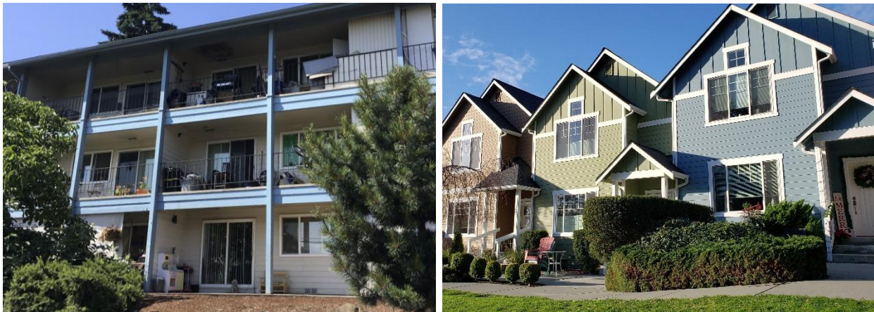
Figure 221. Housing of different designs, ownership arrangements, and prices help meet the diverse needs of Tukwila residents.
