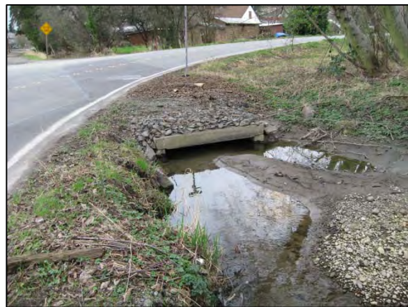
Photo 10. East Fork Southgate Creek: view of the east end of the culvert under 44th Place S (fish passage ID 50016, non-barrier). Flow from the west fork was diverting into a pipe at S 133rd Street, instead of passing into the main channel, due to channel gradient and sediment blockage. (Date: 2/3/2011)
