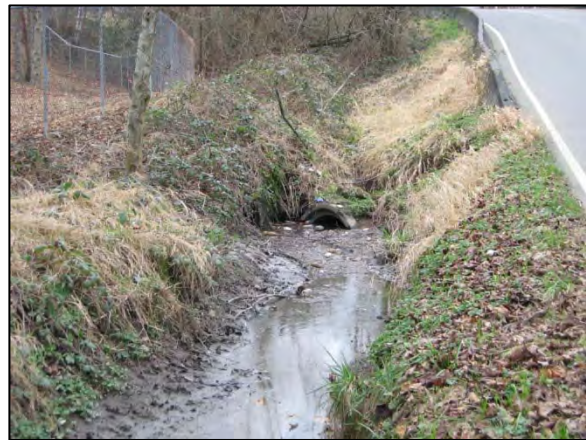
Photo 8. Southgate Creek: view of inlet to City-owned culvert under S 132nd Street (fish passage ID 50015, partial barrier). There was no flow through the culvert due to sediment blockage at the time this photo was taken. (Date: 2/3/2011)
