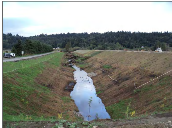
Photo 21. Newly restored section of the main Johnson Creek: reach, looking upstream of the inlet to the outfall to the Green River (fish passage ID 50000, partial barrier). The culvert and flood gate were replaced with a fish-passable structure (passable under most flow conditions) under the mitigation for the adjacent Tukwila South project. (Date: Fall 2011)
