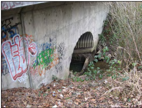
Photo 7. Southgate Creek: view of the outlet of the culvert under Interurban Avenue S (fish passage ID 50013, partial barrier). The fish ladder just inside the culvert is considered a partial fish passage barrier because low flows did not appear sufficient to allow fish to jump over the weirs. (Date: 2/3/2011)
