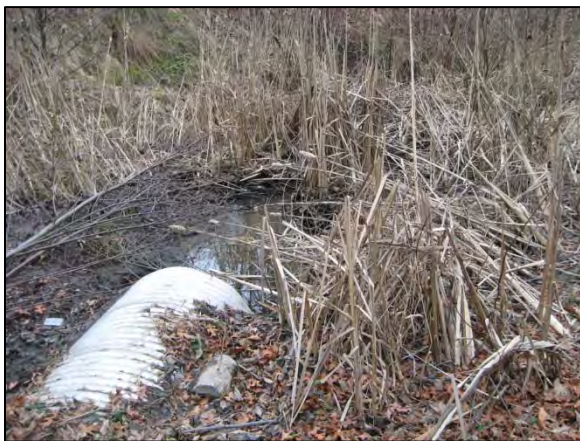
Photo 9. Southgate Creek: view of pipe outlet into the wetland that conveys the main branch (fish passage ID 50015, partial barrier) just upstream of SR 599. (Date: 2/3/2011)
