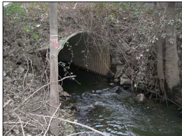
Photo 14. Gilliam Creek: view of the outlet of the WSDOT-owned culvert under the south shoulder of I-405 (fish passage ID 40864, partial barrier). This 1,100-foot long culvert is identified as a partial fish passage barrier likely because of high discharge during high stream flows due to its length. (Date: 2/3/2011)
