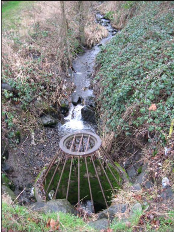
Photo 18. Upper Gilliam Creek: view of the Gilliam Creek RDF structure (fish passage ID 45078, partial barrier). This feature was identified as a partial barrier by WDFW, but appeared to be a total barrier during the windshield survey. (Date: 2/4/11)
