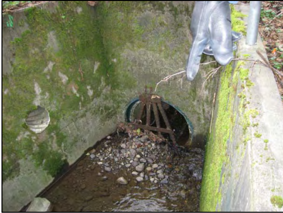
Photo 11. West Fork Southgate Creek: view of the inlet to the long culvert under S 133rd Street (fish passage ID 50021, total barrier). The steep gradient as well as the structures shown here and in Photo 12 combine to act as a total fish passage barrier. (Date: 2/3/2011)
